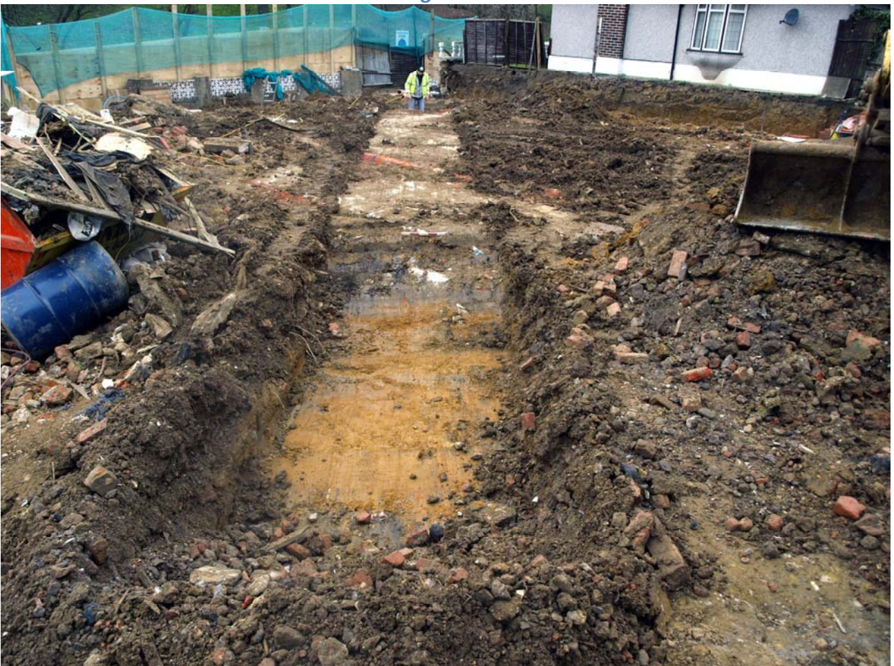
Plate 10: Looking south west at Trench 1 and exposed foundations of demolished house.
