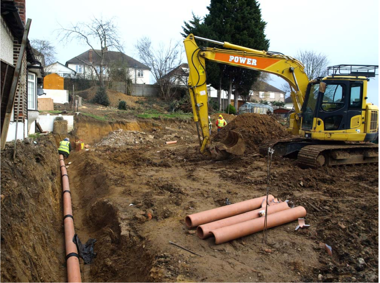
Plate 4: Looking north at trench with laid drain pipe.
