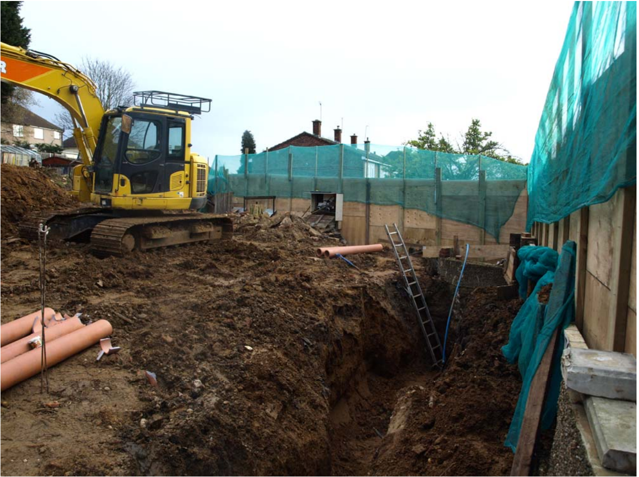
Plate 3: Looking east at trench for drain installation. Trench is cutting through build up terrace. Notice buried fence wall behind the ladder.
