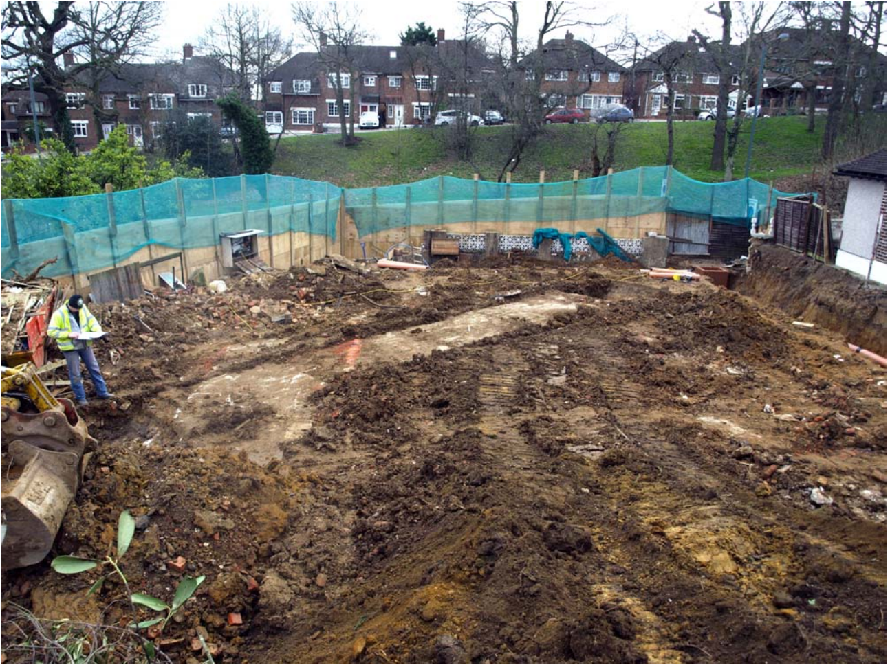
Plate 9: Looking south at Trench 1.
