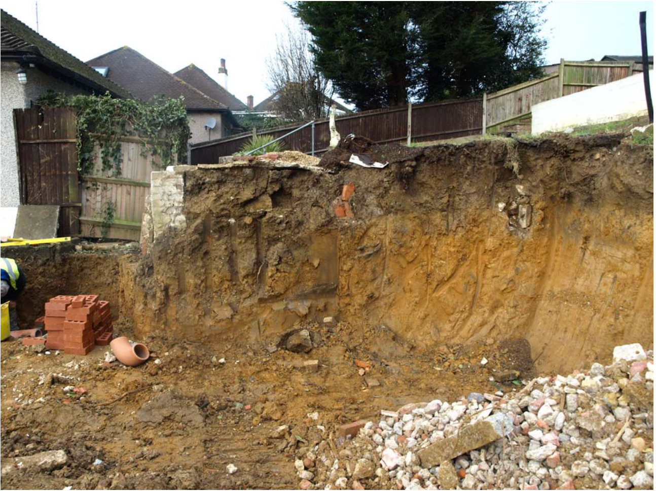
Plate 5: Looking west at scarp exposed after demolition of retaining wall. Two postholes indicating the position of boundary fence are visible in section.
